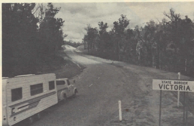
Reconstruction of Princes Highway on new deviation at N.S.W. border.
