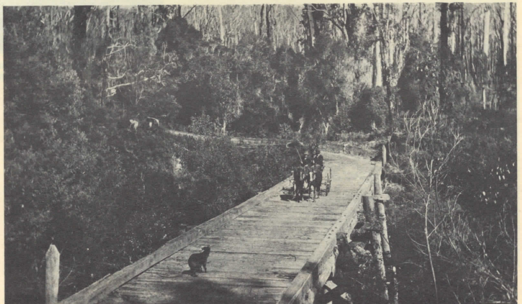
Bridge over Bemm River in 1913.
