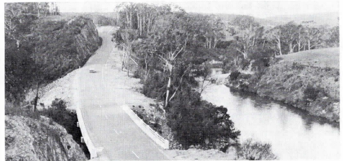
A recently reconstructed section of the Omeo Highway at Monkey Creek, north of Bruthen.
