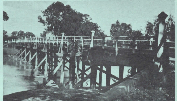
The old Goulburn River bridge which is no longer on the Hume Highway.
