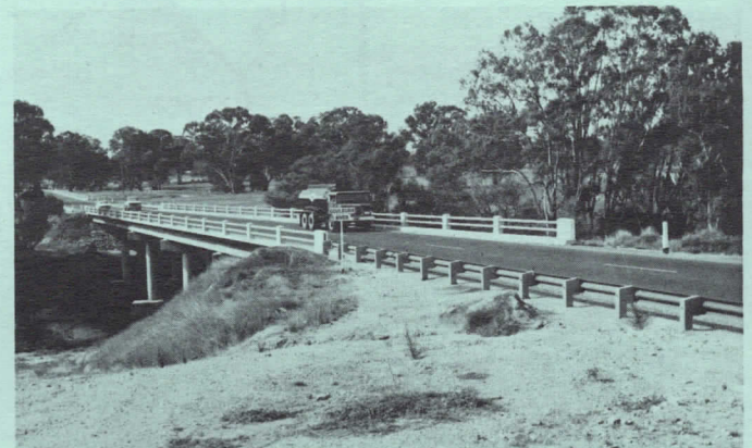
The new bridge over the Goulburn River built on an improved highway alignment.
