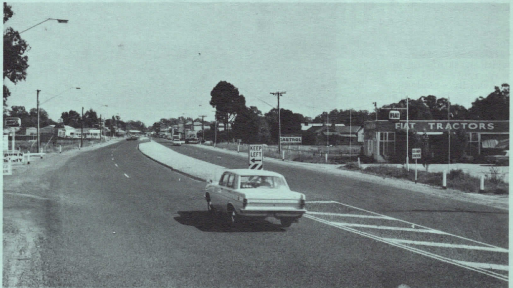
Dual carriageways have now been provided through Seymour.
