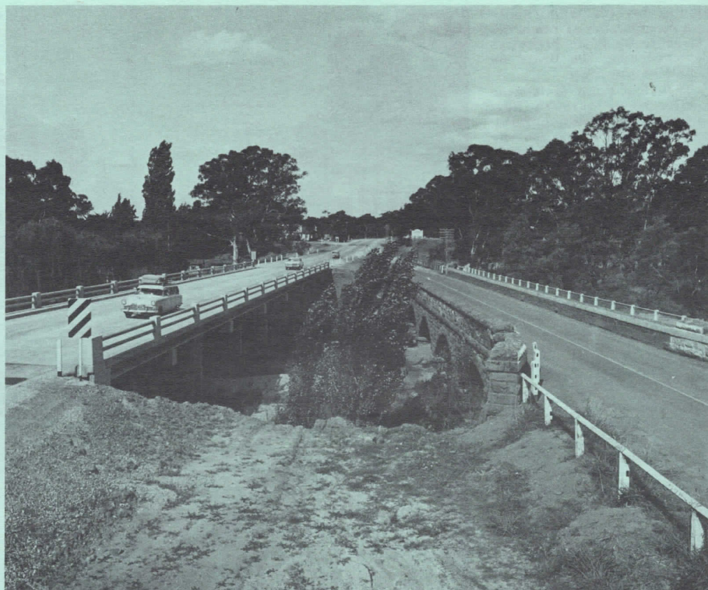
At Avenel the century-old stone arch bridge over Hughes Creek is now only used by pedestrians. Vehicular traffic is carried on a wide, modern, reinforced concrete bridge.
