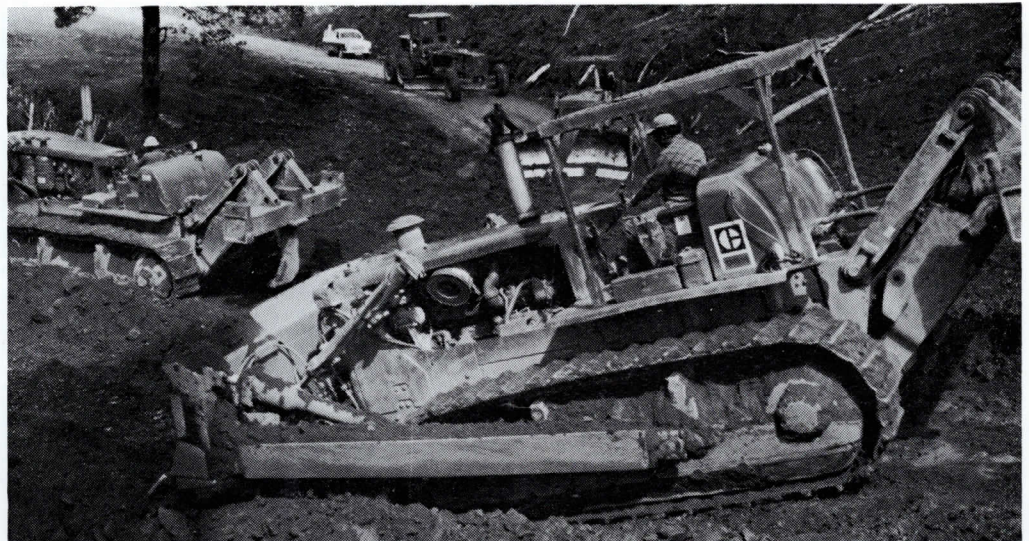
Reconstruction of the Ocean Road in progress south of Lavers Hill.
