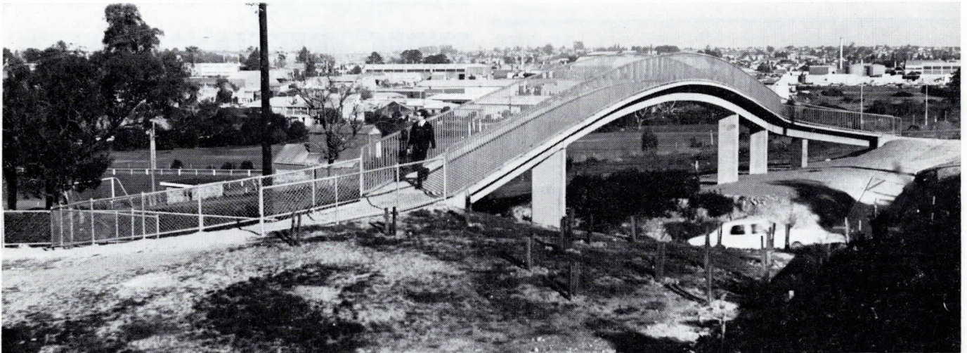
Pedestrian overpass, Canterbury Road, Box Hill South.
