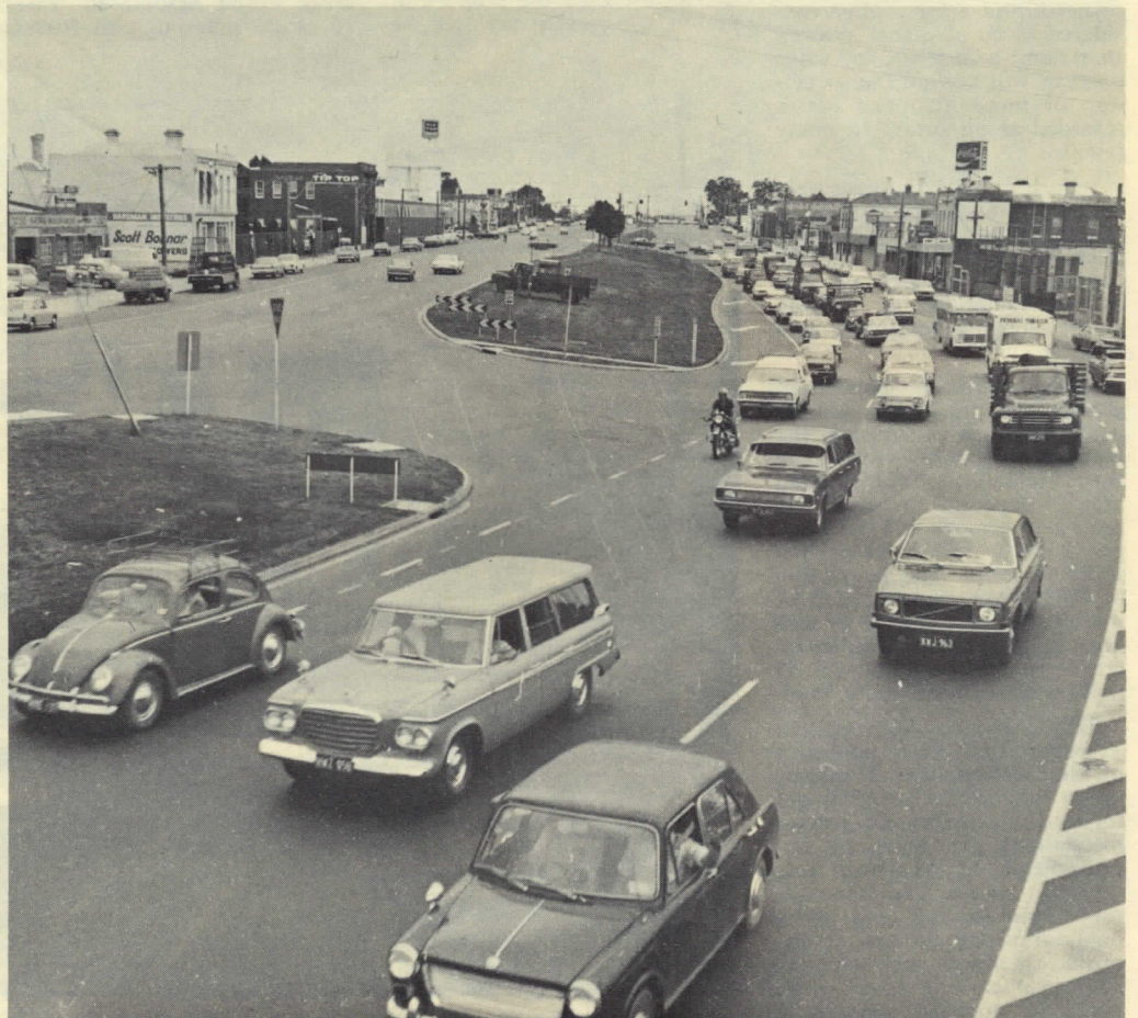
Dual carriageways each of three lanes have been provided for through traffic on the Princes Highway at Oakleigh.
