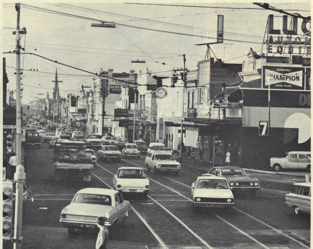
Sydney Road, Brunswick — traffic congestion because of inadequate road width, frequent intersections and adjacent commercial development.
