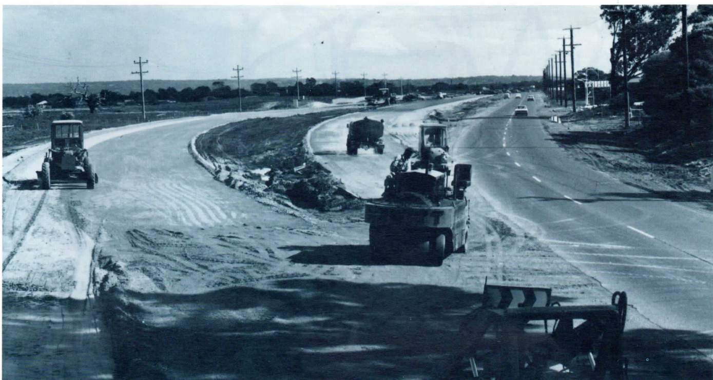
Work in progress on the Frankston Freeway near Armstrongs Road, Seaford.
