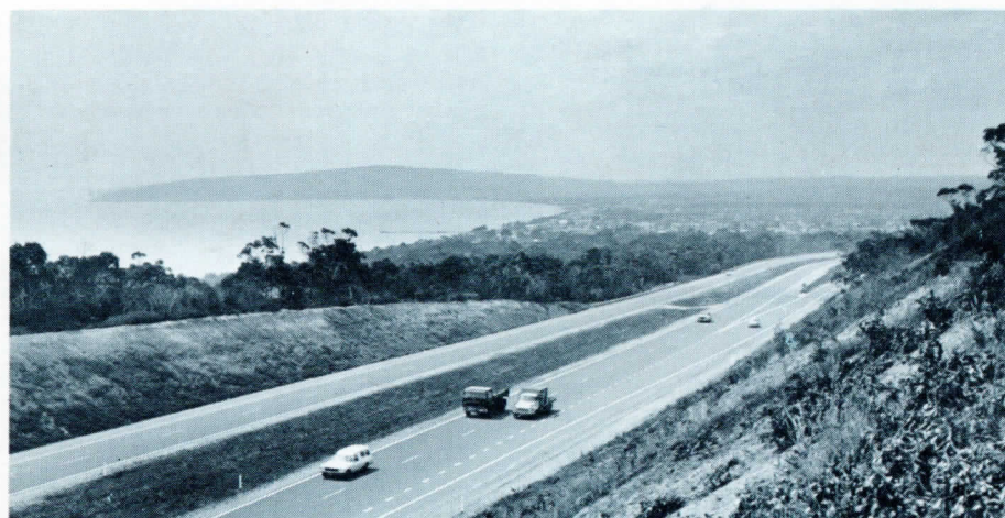
The Mornington Peninsula Freeway — one of the major C.R.B. projects which will be continued in 1973/74.
