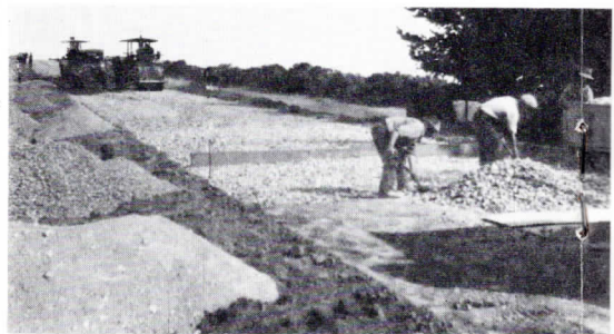
● 1930... spreading base course at Burrumbeet.
