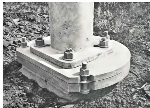
Slip Based Light Pole Anchorage
