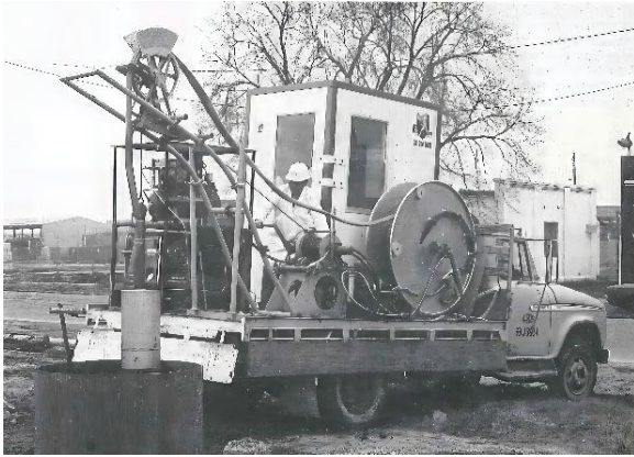
Lowering SID into the cylindrical pile casing
