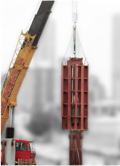
20-tonne hammer dropping onto pile
