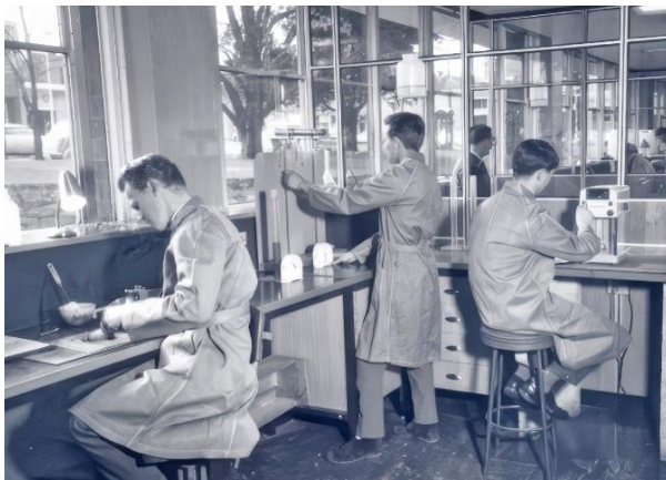
Soils staff undertaking PI and Sand Equivalent testing
