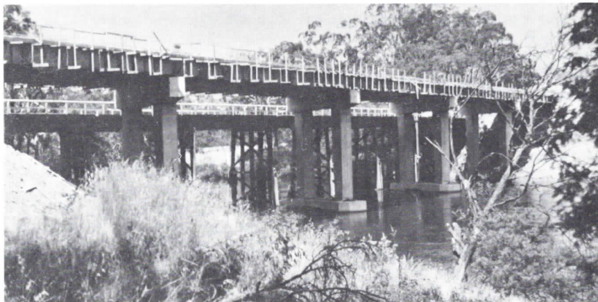
Construction of a new bridge to carry the Goulburn Valley Highway across the Goulburn River at Trawool will be completed in May 1977. The five span bridge and roadworks is estimated to cost $1 million.
