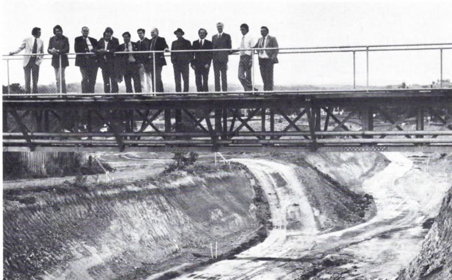
Some of the conference delegates inspect work on the Greensborough Freeway site where road over rail overpasses are being constructed.
