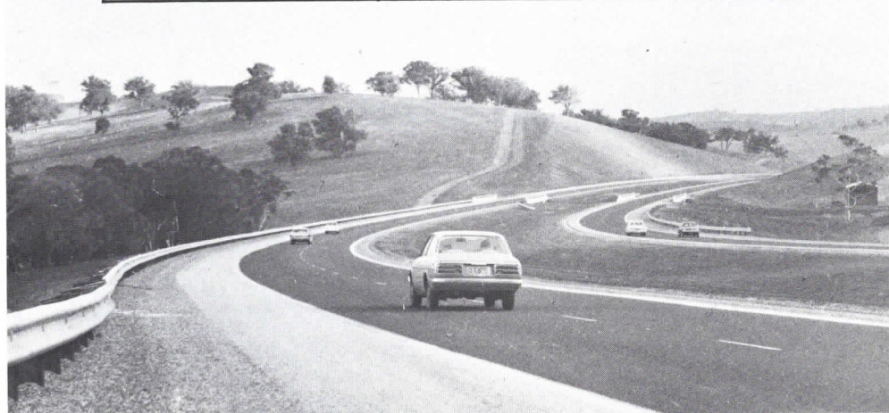
TOP: Trees, shrubs and ground cover planted as part of the landscaping treatment on the Mulgrave Freeway, Doveton.
