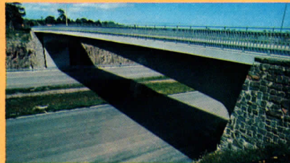
● The National Park overpass on the Yarra Bend Park Road.
