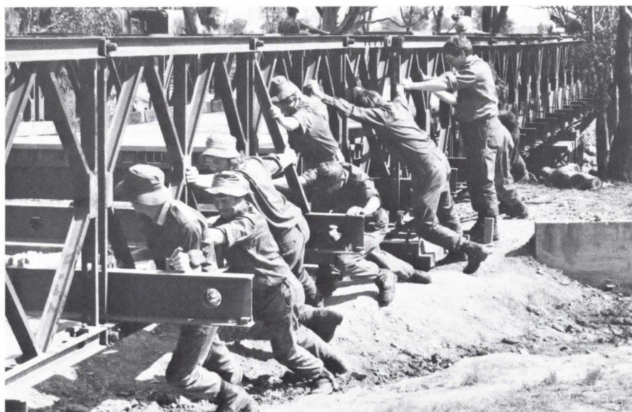
● Army reservists from the CRB construct a Bailey Bridge during training. Volunteers with the Supplementary Reserve attend a two-week camp each year.
