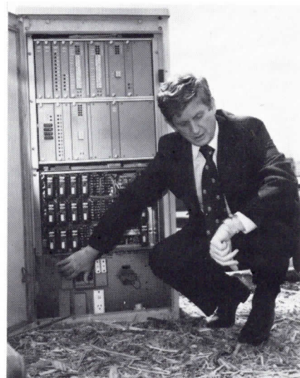
● Mr Maclellan turns off the last set of traffic signals on the Tullamarine Freeway — right on time.
