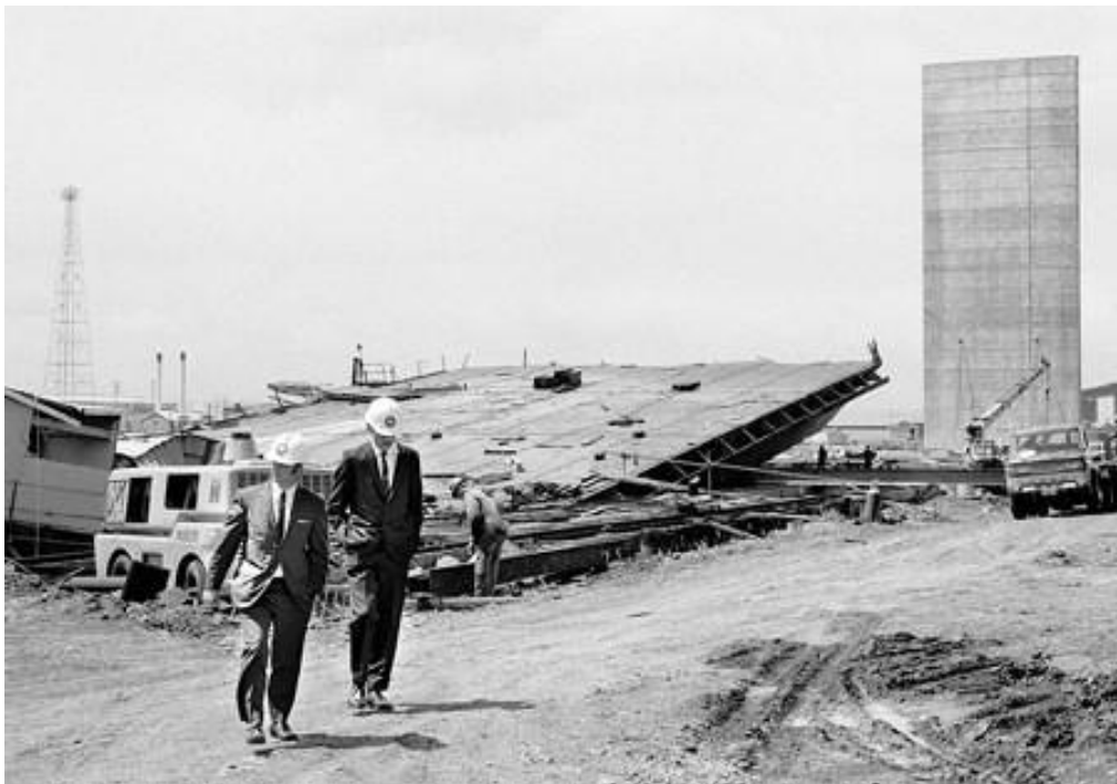
The fallen span, with Pier 12 in the distance. (Image courtesy of Rob Morgan ARPS)
