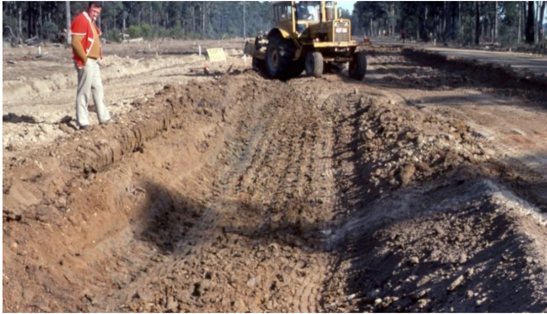
Overseer Sandy checking for soft material on the Simpsons Creek project
