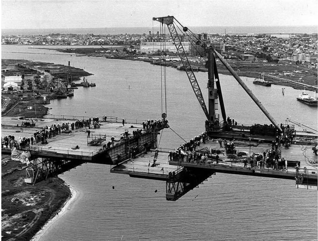
Figure 1- The final box being erected in May 1978
