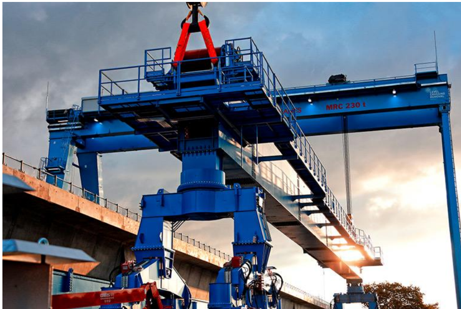
A 60m wheeled straddle carrier in action at Murrumbeena, installing its first piece of elevated rail.
