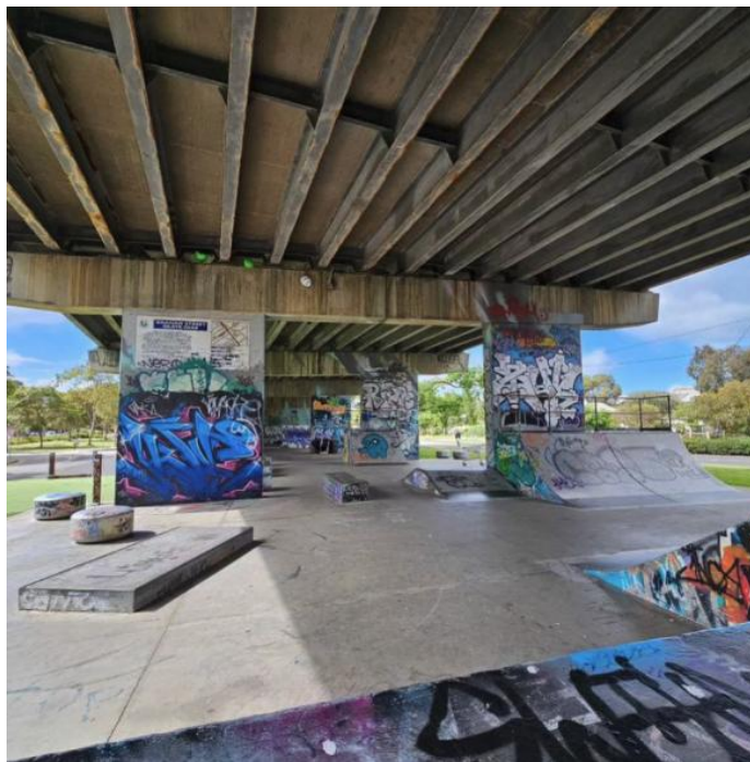
Graham Street railway overpass – now converted to a skate park. The graffiti and skateboard ramps were not included in the project.
