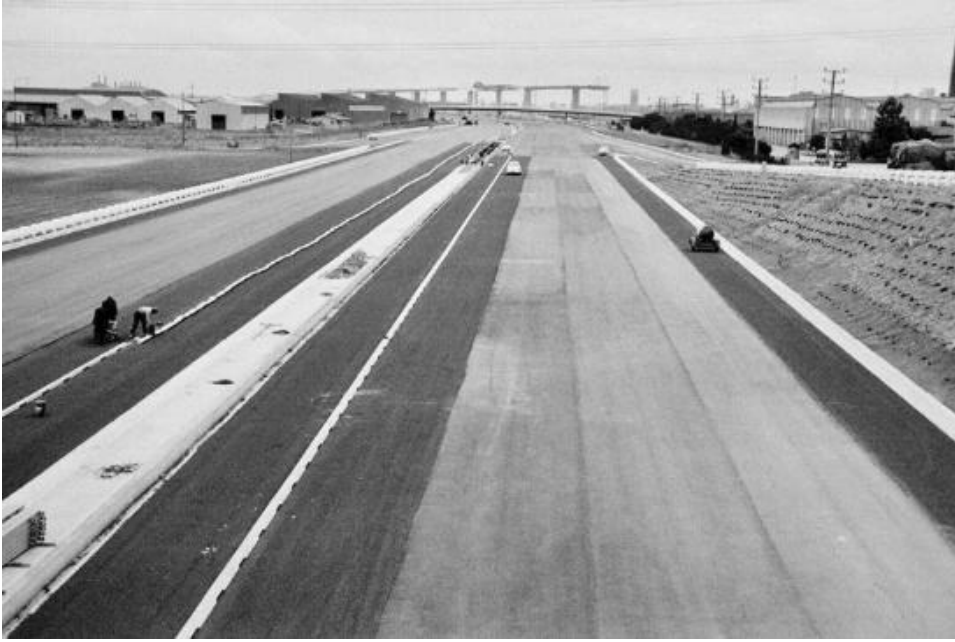
Looking west along the Lower Yarra Freeway from the Graham Street overpass (now the M2 Citylink interchange bridge), late October 1970. (Image courtesy of Rob Morgan ARPS)
