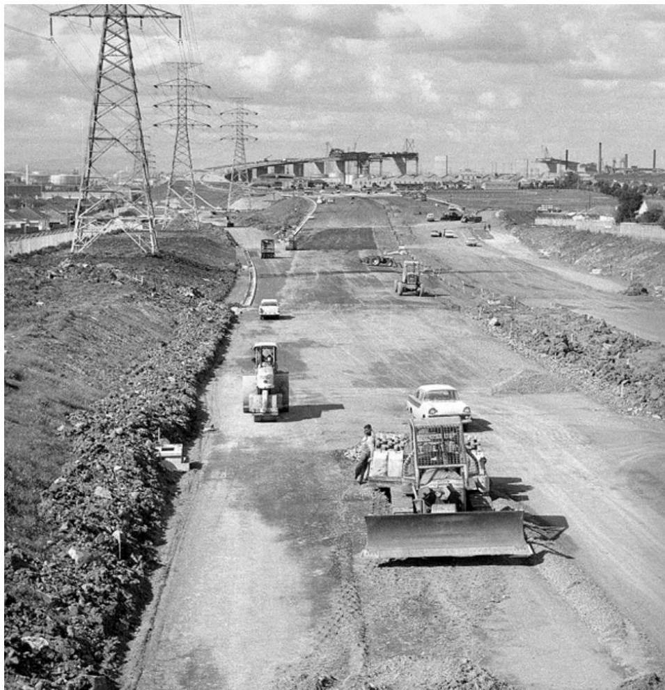
The Lower Yarra Freeway under construction in August 1970 looking east from the Wembley Avenue pedestrian overpass towards West Gate Bridge. (Image courtesy of Rob Morgan ARPS)
