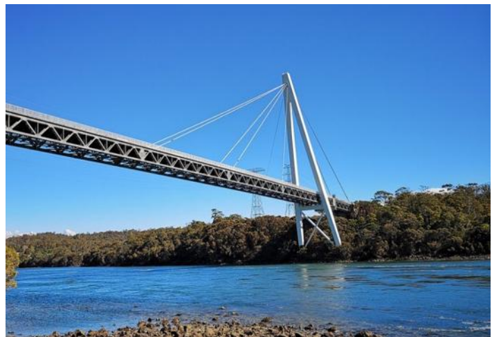
Batman Bridge, Tasmania
