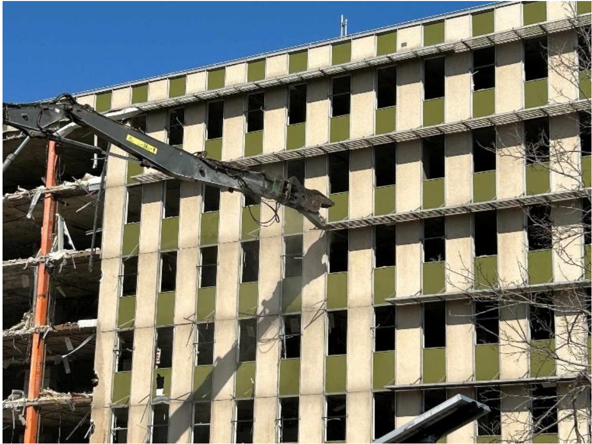
This picture of the building's northern face was taken on 2 September. It shows a specialised wrecking machine plucking off the aluminium sunshades. The same machine was used to remove the concrete panels at the left of the picture.
