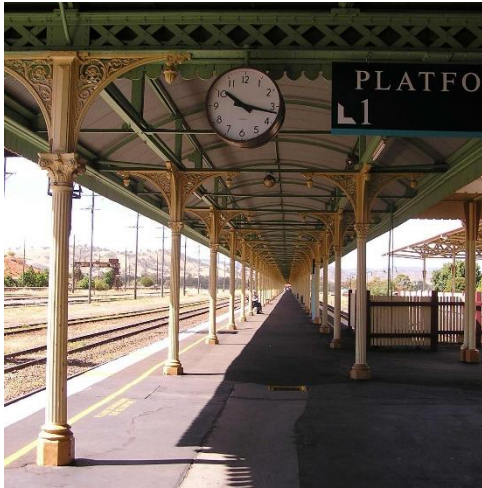
The transfer platform at Albury Station. The standard gauge is on the left; broad gauge on the right
